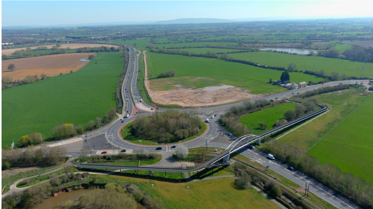
Figure 2-4 - Overview of Powick Roundabout post Completion
