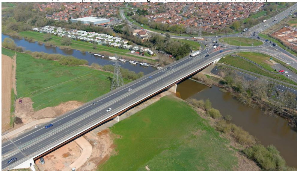
A4440 SLR4 Improvements (Looking north towards Powick Roundabout)
