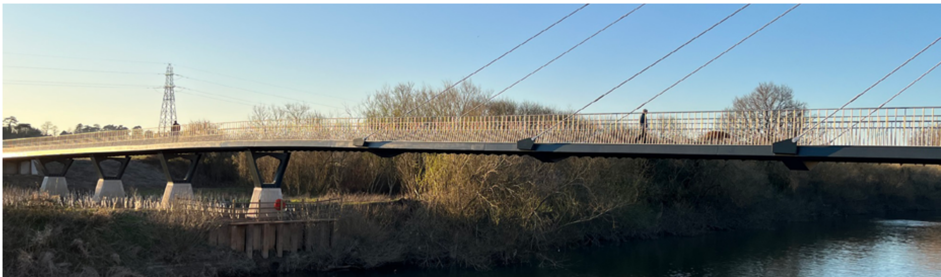
Kepax Bridge, Worcester
